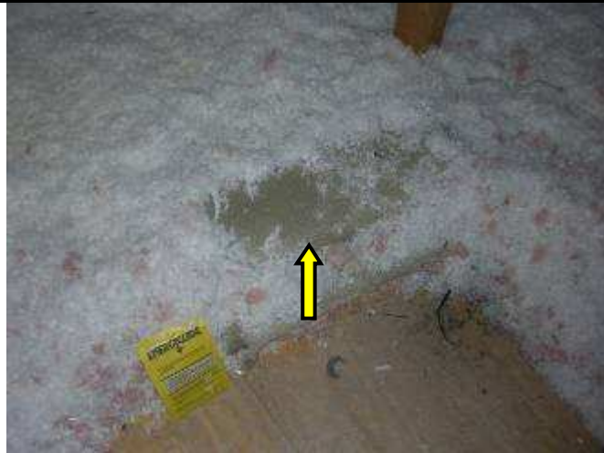
Carpet in insulation
