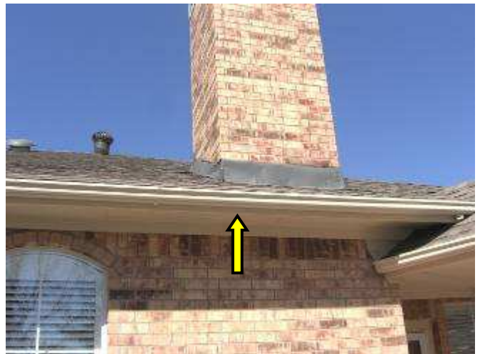
Loose gutter
