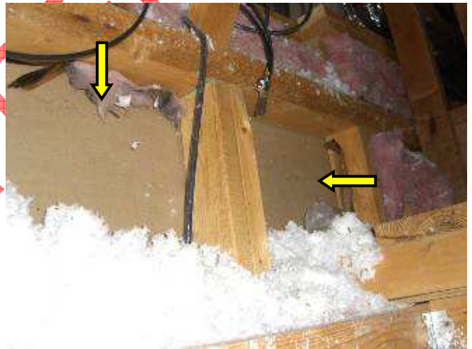
Missing insulation
