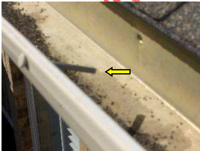
Broken fastener
