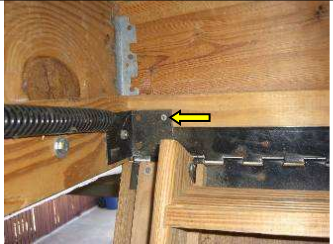
Incorrect fasteners
